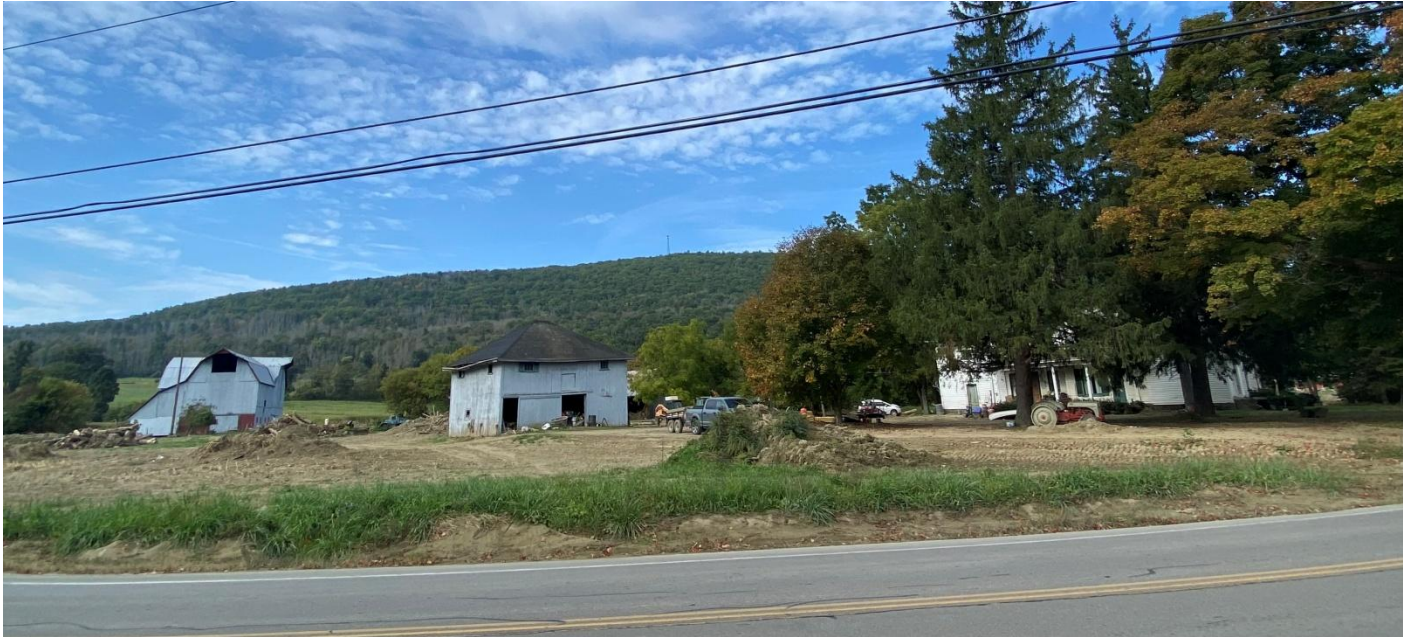
Willow Bend Barn after August 9, 2024 Flood
